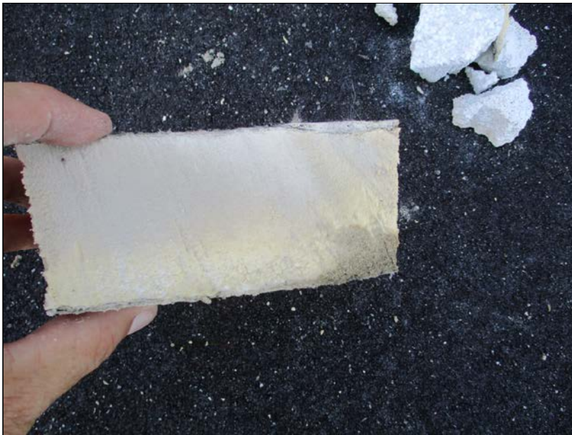
Photo 4: Core location C6, nuke reading 6 – polyiso insulation.
