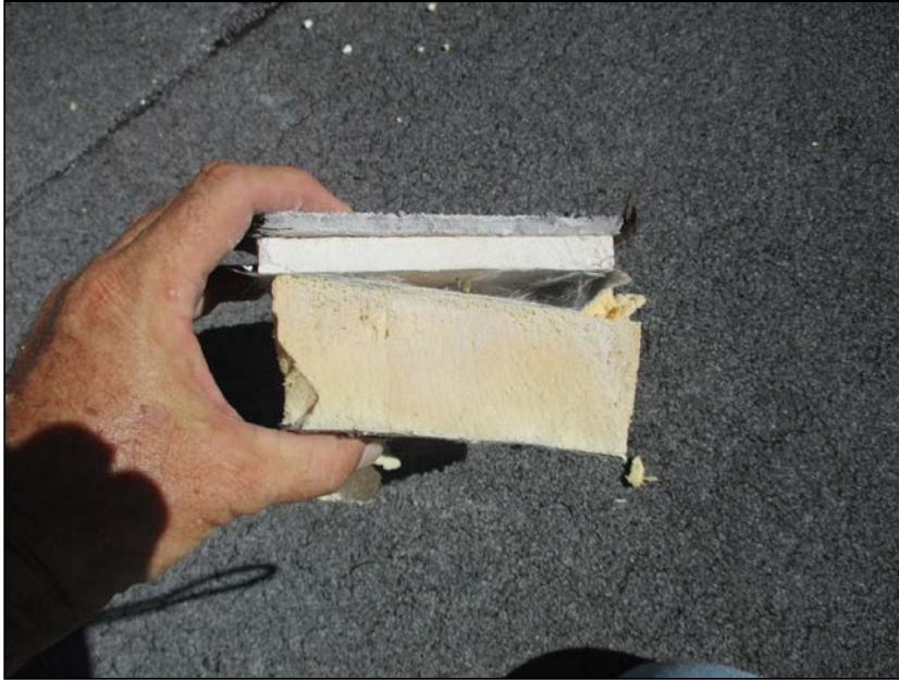
Photo 5: Core location AC5, nuke reading 8 – relatively dry roof components.
